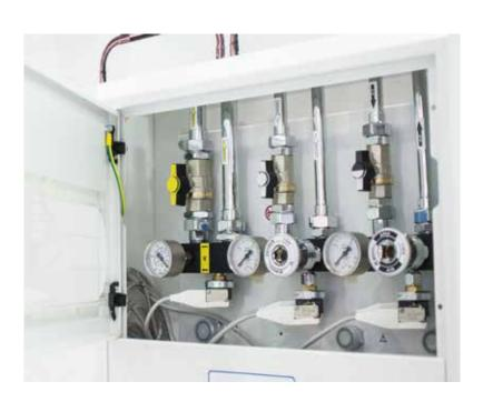
AVSUs are installed in each operating room, ICUs, resuscitation rooms and in other hospital areas. AVSU are equipped with a lock that can be opened with a key and as reccomemended in ISO 7396-1 (Medical gas compressed pipeline systems and vacuum) can be opened by a special system in case of emergency.
